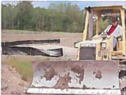
Silt fencing on-site
