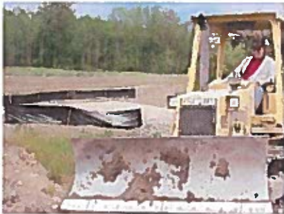
Silt fencing on-site
